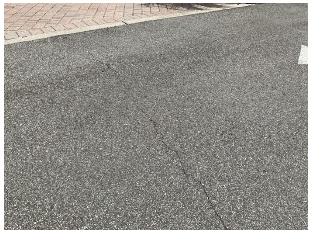
Pavement cracks at the Clubhouse parking lot area
