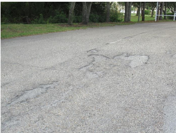
Cracked pavement and deterioration at the entrance
