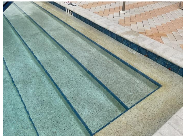
Pool plaster finish with tile perimeter
