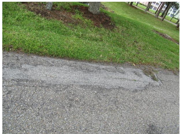
Pavement deterioration and pothole formation
