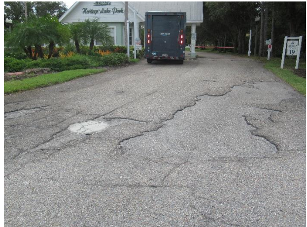
Cracked pavement and deterioration at the entrance
