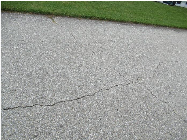
Pavement cracks
