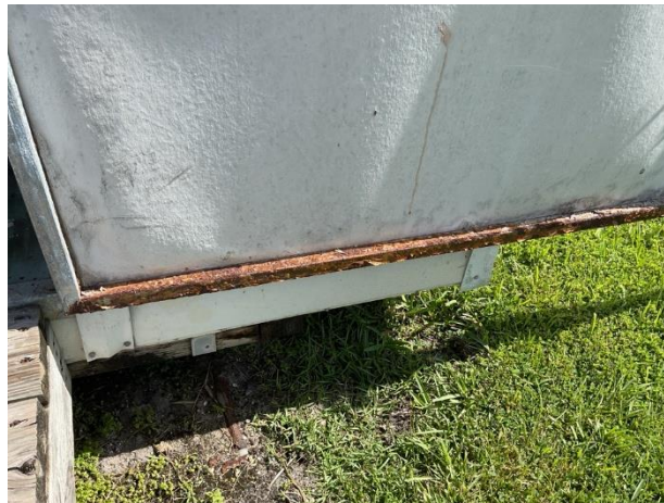
Rust formation on the exterior door
