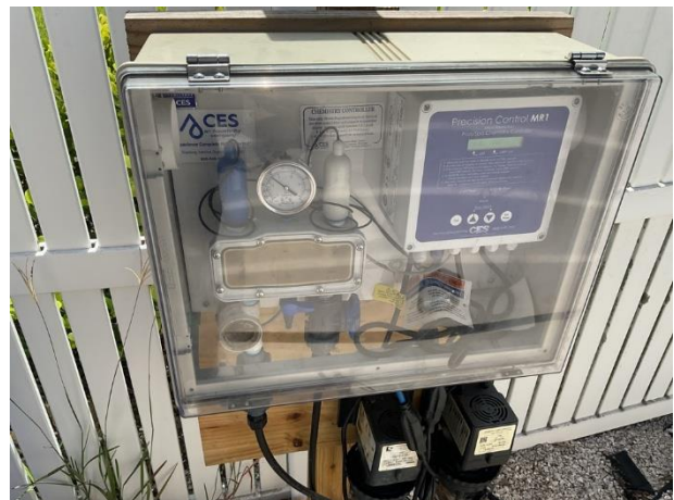
Automatic chlorinators and controls
